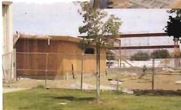
Wellness center under construction
