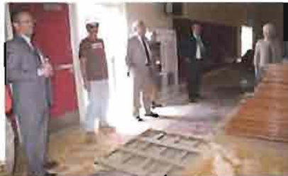
Administrators and board members tour the gymnasium while renovations are underway
